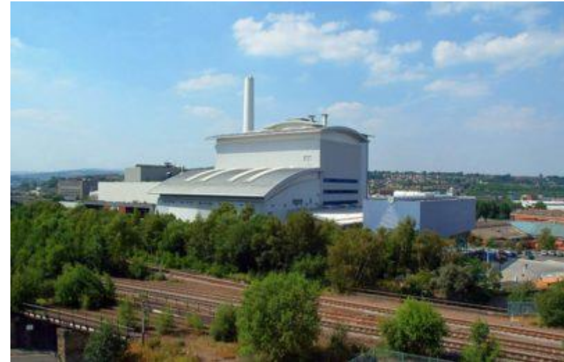
Veolia Energy Recovery Facility; Bernard Road, Sheffield.
