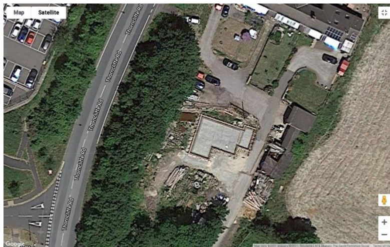
Dwelling Under Construction Planning 16/00800
