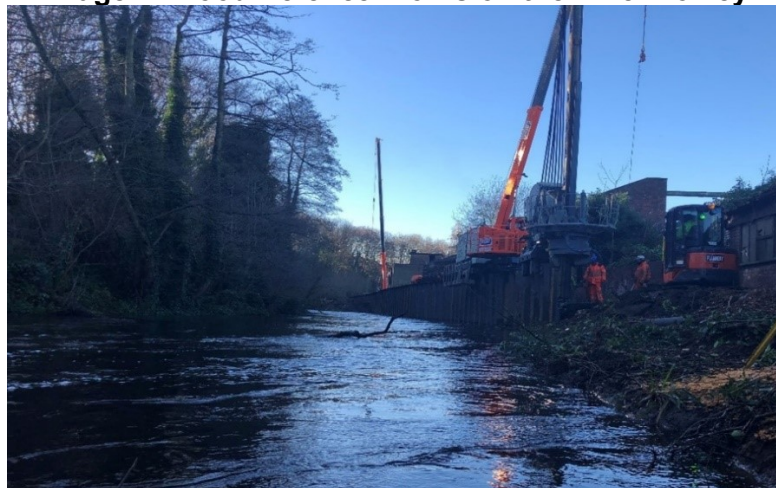
Image 1: Flood Defence Works on the River Loxley
